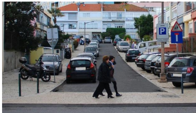
Figure 20 – Continuous sidewalk (EPAP, 2014b)
